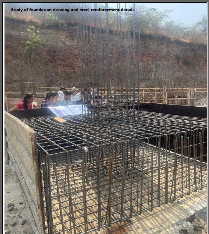
Visit to Polytechnic building site on 27/03/2025
